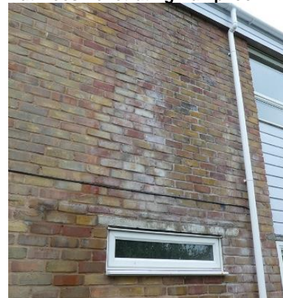
What Does Defective Plumbing Damp look like?
